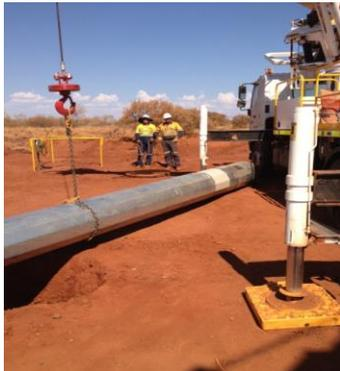
Lost control of load – Rigging method incorrect. Changes to the planned lifting / rigging method and equipment were not authorised and there was inadequate competent supervision of a complex lift.
